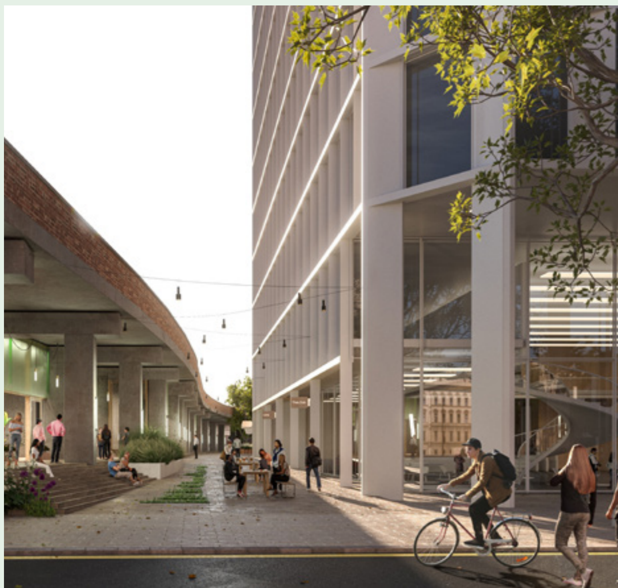
Illustrative view from Upper Marsh looking towards the Low Line with the renovated railway arches
